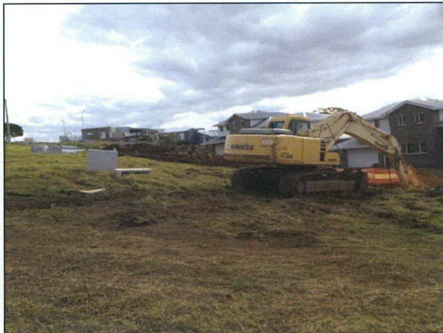
Plate 4: View of medium residential development to west of subject site.
